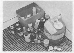
CHEMICAL WASTES, separated in bays by category, are placed on grates over open concrete sumps. Therefore, if a container leaks, the spillage is contained within the facility.
